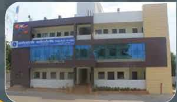
3PL Admin Building
