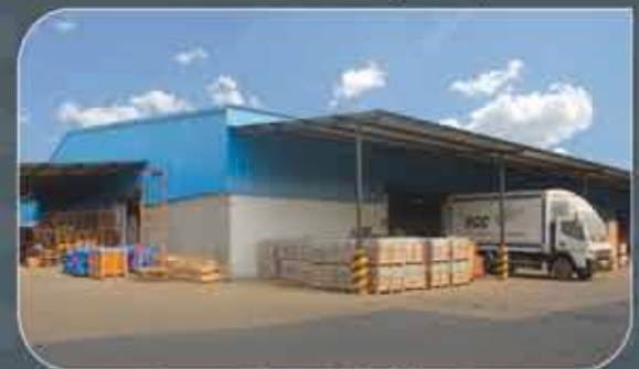
Covered Carting & Stuffing Area
