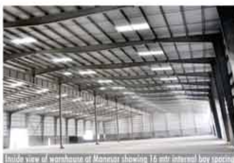
Inside view of warehouse at Manesar showing 16 mtr interval bay spacing
