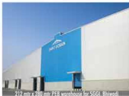
212 mtr x 280 mtr PEB warehouse for SGGI Bhiwadi
