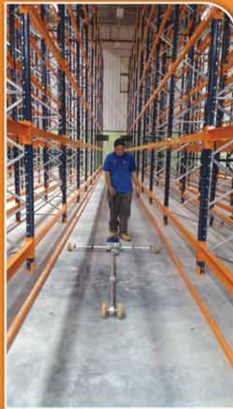
SUPERFLAT FLOOR SURVEY
