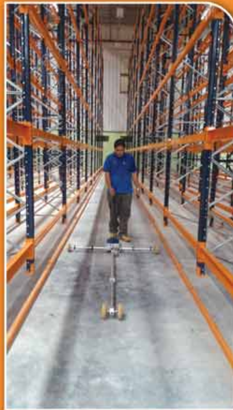
SUPERFLAT FLOOR SURVEY
