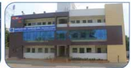
3PL Admin Building
