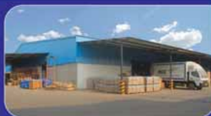
Covered Carting & Stuffing Area
