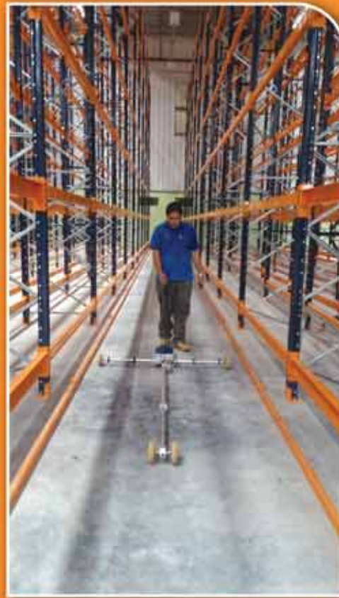
SUPERFLAT FLOOR SURVEY
