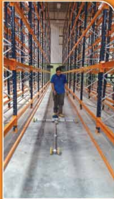
SUPERFLAT FLOOR SURVEY
