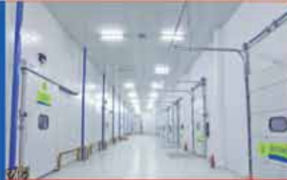
Temperature Control Handling Area
