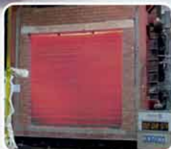
AFTER 2 hrs FIRE TESTING
