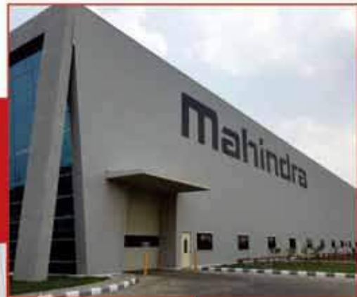
State of the art, 10,000 sq.mtr. Industrial facility for Mahindra Auto Steel, Pune
