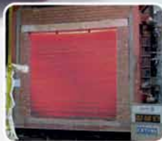
AFTER 2 hrs FIRE TESTING
