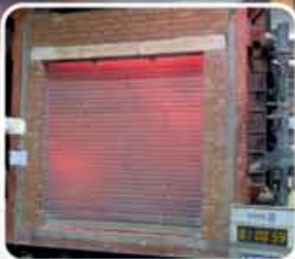
AFTER 1 hr FIRE TESTING
