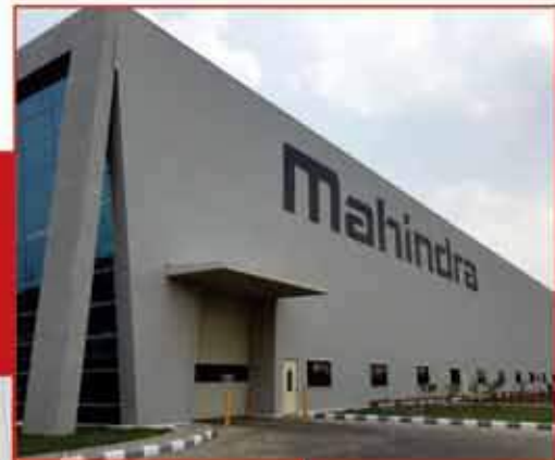
State of the art, 10,000 sq.mtr. Industrial facility for Mahindra Auto Steel, Pune
